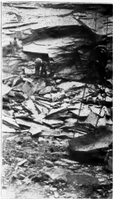
Removing Good Material After Small Blast.
